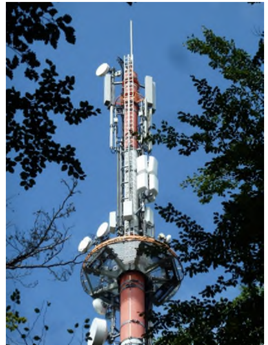
picture 1, right: Transmitting site "Leonberg" with new circular polarised KATHREIN UHF antennas
