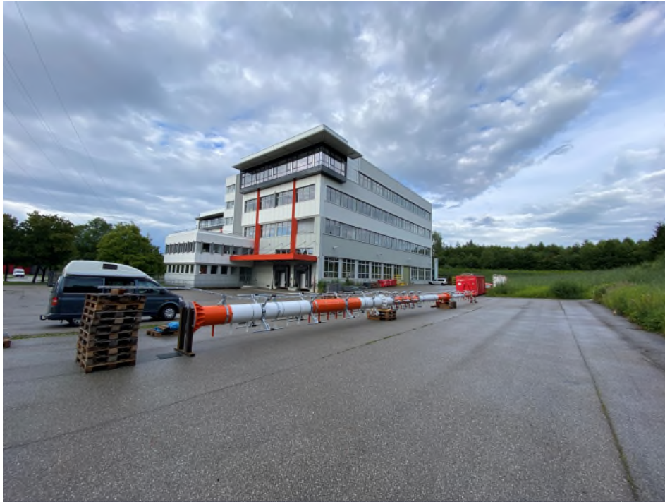
Final assembly of the 26 meter long antenna in the courtyard
