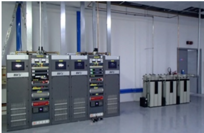
Picture 1, left: Transmitter room with KATHREIN FM Combiner
