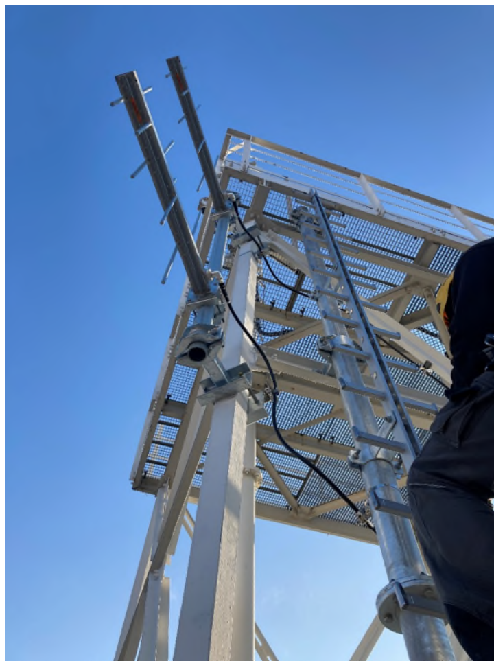
picture 1, above 2 vertical polarised KATHREIN Log. Per. Antennas ensure DAB+ reception
