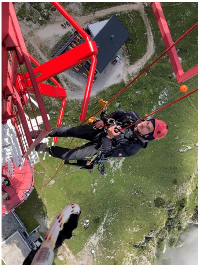
picture 2, left: Rigger at a lofty height when replacing the antennas
