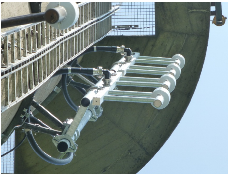
picture 1, above: The DAB+ transmitting antenna with four vertical dipoles
