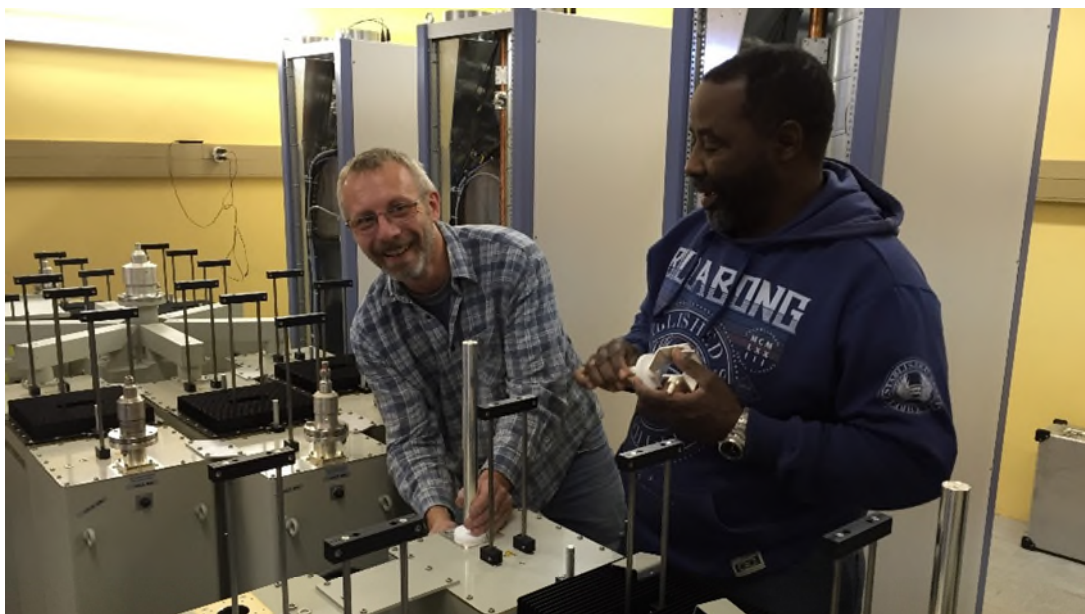
Left picture: Gerhard Lerche (Kathrein, left) and Mbeno Murangi (NBC, right) tuning a FM combiner.
