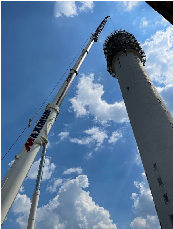
picture 2, above: A mobile heavy-duty special crane with extension boom lifts the antenna system on the top of the concrete tower
