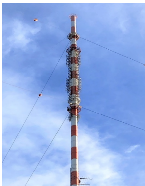
picture 2, left: The DAB+ antenna is at the top in the GRP cylinder
